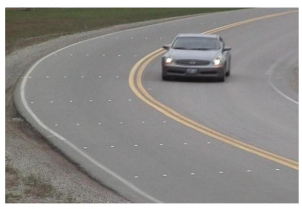
The road in question was signed with a maximum posted speed of 80 km/h. The curve a itself was posted with an advisory speed of 60 km/h. Yet the average speed of vehicles entering the curve was 79 km/h and exiting at 75 km/h; both well above the advised speed.
